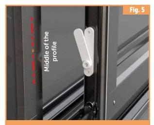
Mark this position and pre-drill a hole with a diameter of 3.5 mm and then 5.5 mm to a
